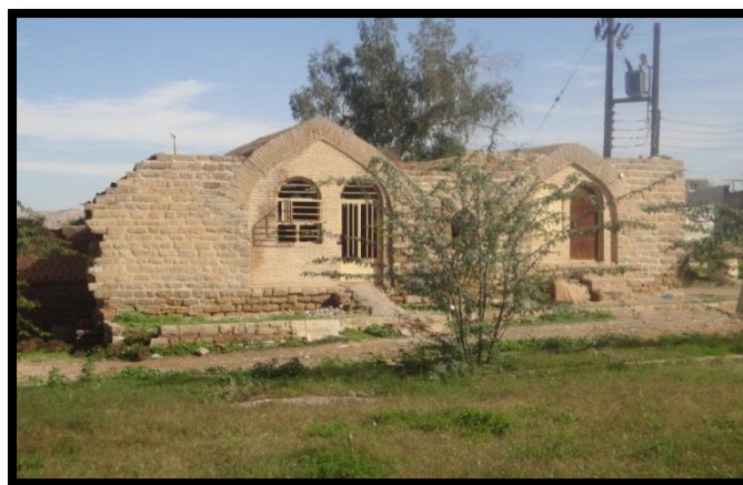
Figure 4: Non-normative restoration of Shadorvan dom-bridge, 2013. Source: Fereshteh Tleb-Mashhadi.
