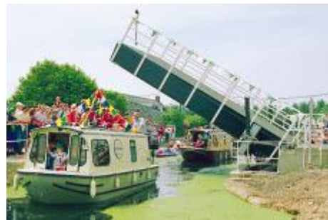
Bonds Mill Lifting Bridge
